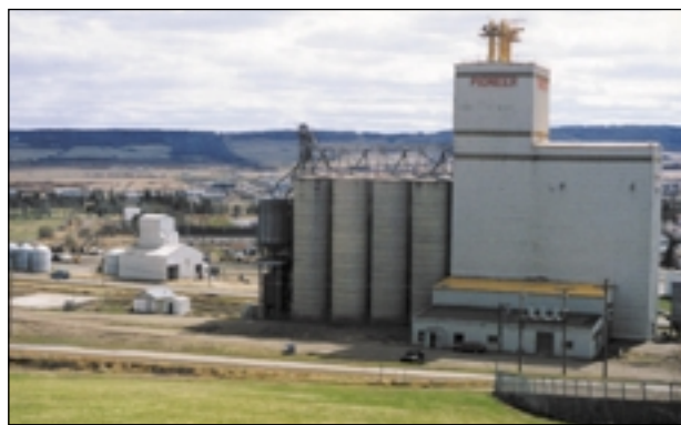
A granary in Peace River, where 35% of farm receipts are generated from grain and oil seed production.
