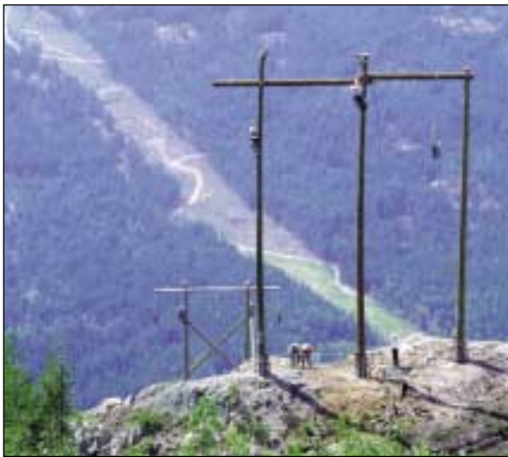
Construction of transmission line for Arrow Lakes Generating Station
