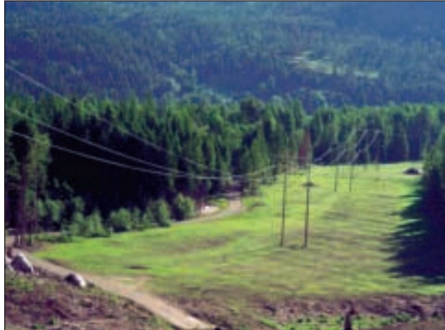
Power transmission lines from the Arrow Lakes Generating Station
