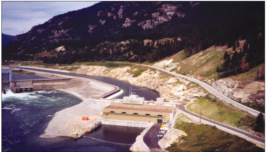
Arrow Lakes Generating Station
