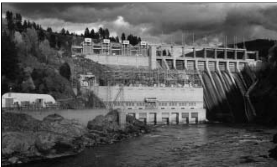
Waneta Dam, owned by Cominco Ltd., is located on the Pend d'Oreille River just upstream from where it joins the Columbia River.
