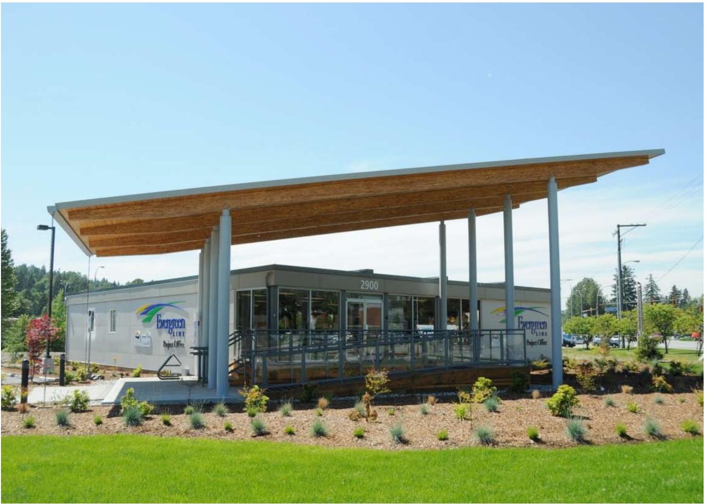
Evergreen Line Project Office, Coquitlam
