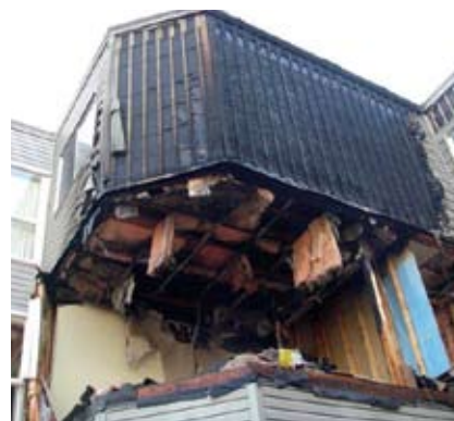
Smart meters will decrease illegal electricity diversion (shown here), keeping neighbourhoods safe from fires like the one that destroyed this house.
