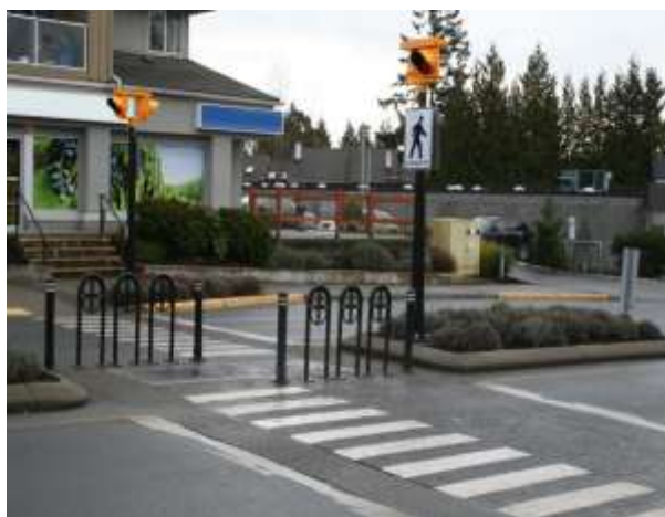
Many countermeasures help protect pedestrians. For example, Danish Offsets at the middle of a multilane crossing provide refuge for pedestrians and ensure they are facing the traffic before crossing the second half of the roadway. Danish Offset Crossing. Photo credit: David Coburn, Neil Arason.
