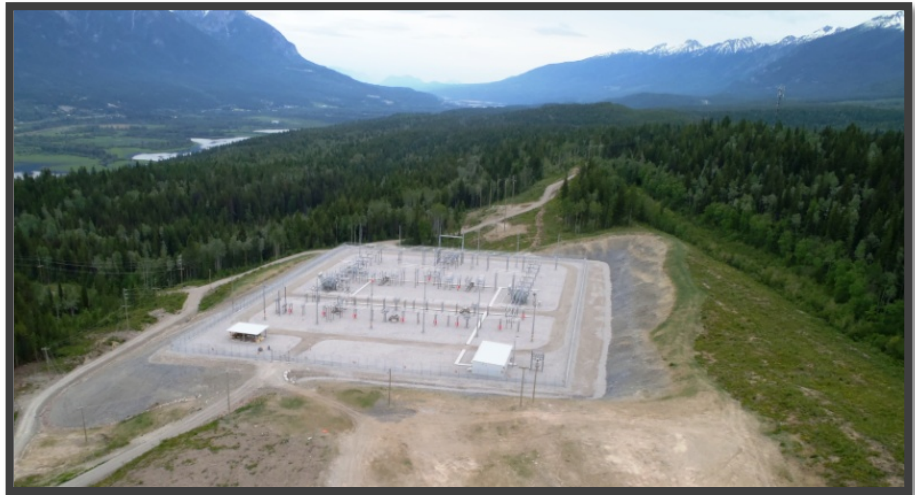
Kicking Horse substation, west of Golden, BC and the Columbia Valley transmission line extending south towards Invermere.
