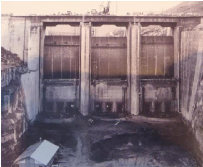
W.A.C. Bennett Dam spillway during original construction in the 1960s, showing the upstream side of the three large spillway operating gates, as well as the nine sluiceways located underneath.
