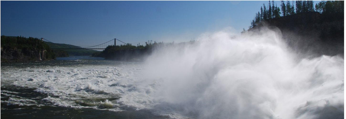
A spill at the Peace Canyon Dam, located next to the Peace Canyon Generating Station.
