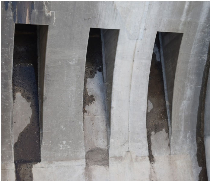
Seen from above, three sluiceways at W.A.C. Bennett Dam.
