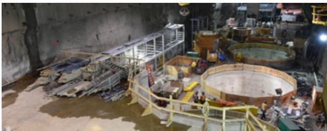
View inside the John Hart powerhouse cavern – 10 stories high – where three new turbines/generators and a water bypass facility are being constructed.
