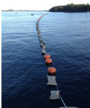
New cable floated from barge using airbags, near Ahousaht, and then directed to underground ducts by divers.
