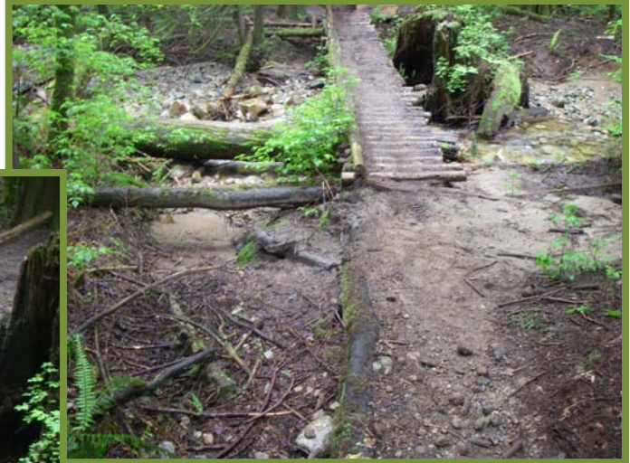
Trail approach to walkway introduces silt and soil to Kathryn Creek.
